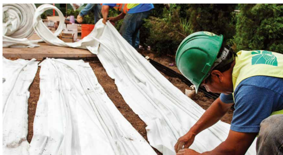
Eco-Mat instalado
